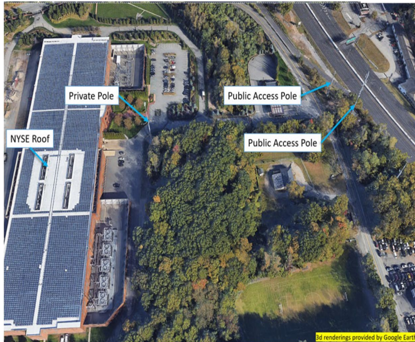
Figure 4: Mahwah Data Center 1
